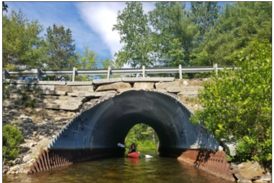
The Tenny River Culvert under Route 85 (Shannon Bryan photo)
